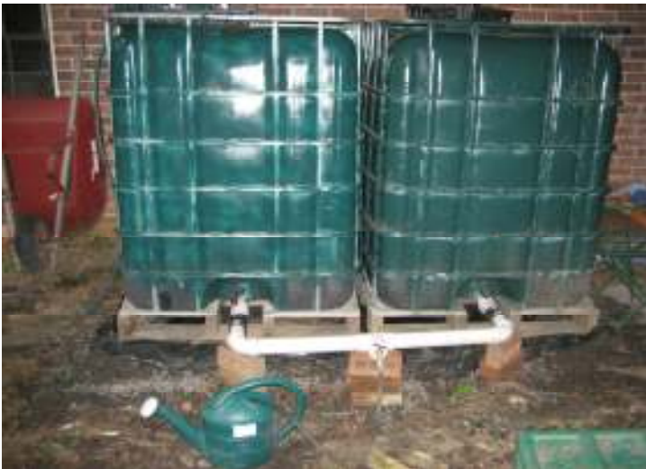
TWO 340 GAL WATER TANKS UNDER JOHN KREINER'S DECK
